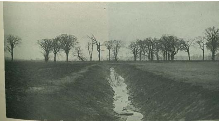
A section of a municipal drain. Raw banks contribute large amounts of silt which finds its way into ponds and the main stream.
