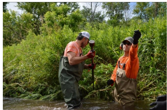
5 / 6 Two volunteers anchor Christmas trees to the river bank to reduce erosion and create fish habitat. Photo
