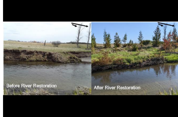
3 / 6 Before and after river restoration. Images supplied by the Nottawasaga Valley Conservation Authority
