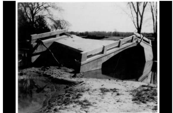
4 / 7 Hurricane Hazel caused extensive damage in 1954.Photo supplied by the Nottawasaga Valley Conservation Authority
