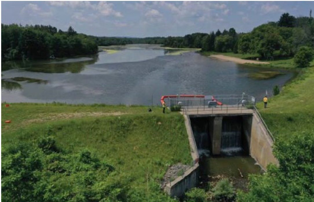
Figure 3. New Lowell Dam and reservoir during summer operations, with the public safety boom in place upstream of the concrete control structure (credit: D.M. Wills, July 5 2023).
