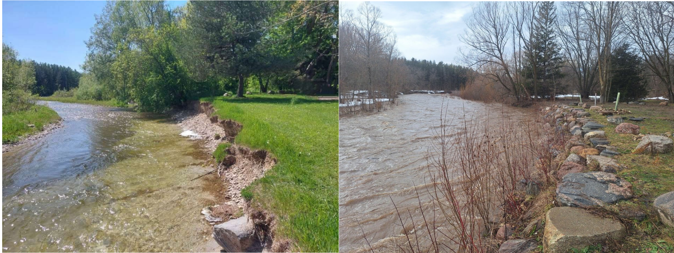
Figure 2a (left): Pre-restoration erosion and undercutting along the Mad River in a Township of Clearview municipal park adjacent to park access. Figure 2b (right): Post-restoration bank treatment reducing erosion risks to municipal infrastructure.
